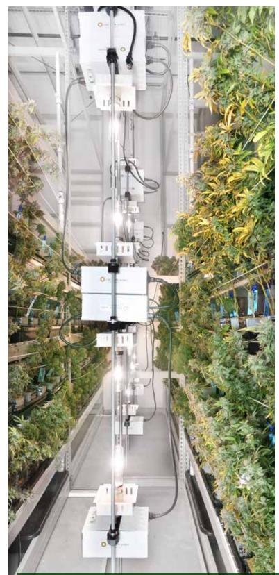
PortaFab's structural framing systems allow for self supported structures up to 24' tall allowing for integrated racking systems.
